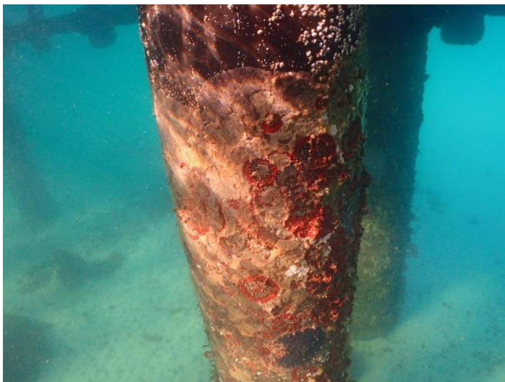
Figure 14. New lower landing HDPE jacketed steel piles: upper section of pile
