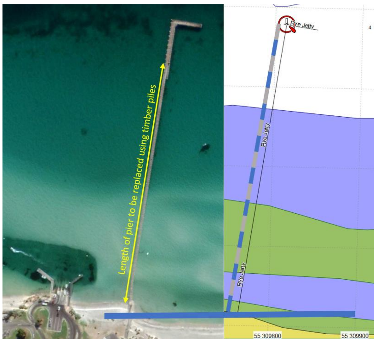
Figure 1. Rye Pier showing length to be rebuilt and bathymetry (Blue and grey bars on right-hand figure are approximately 20 m intervals)
