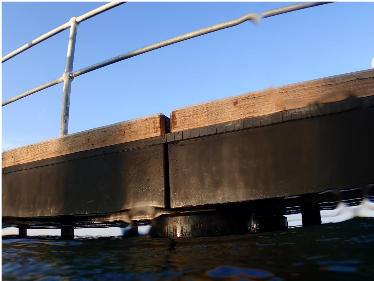
Figure 13. New lower landing Rye Pier July 2021
