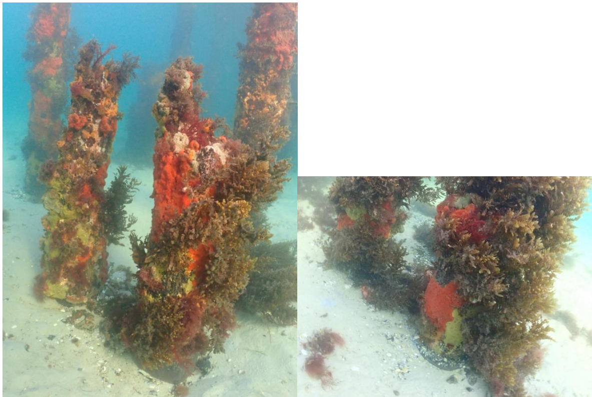
Chainage 200, SD 2.8 m, CD 1.9 m Chainage 220, SD 3.0 m, CD 2.1 m Figure 7. Pier piles chainage 200 and 220
