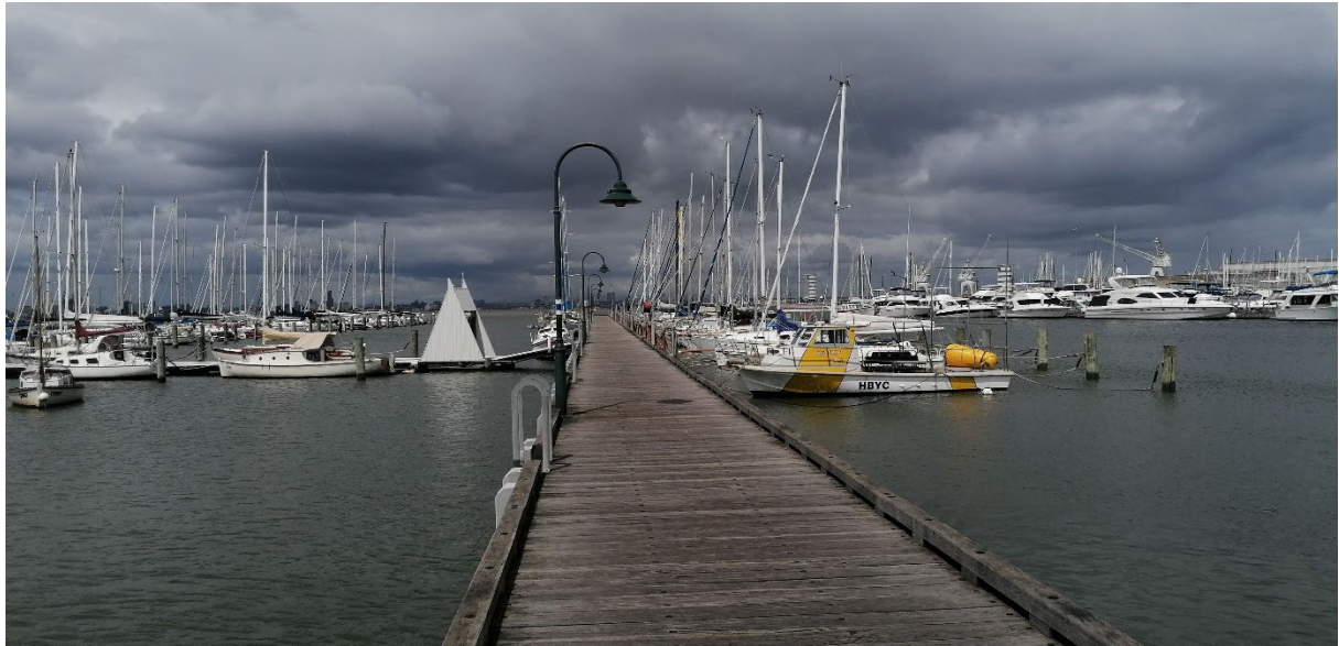
Figure 19. View along the timber deck section of Ferguson Street Pier with public moorings (right) and Hobson's Bay Yacht Club marina (left).
