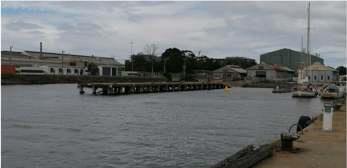
Figure 22. Boyd Street Pier viewed from Workshops Pier.
