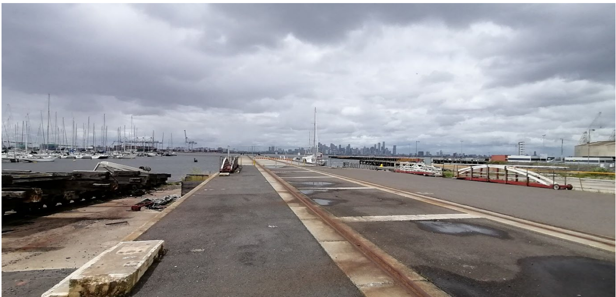
Figure 26. The main deck of Workshops Pier looking towards the city of Melbourne. (Source: GML 2022)
